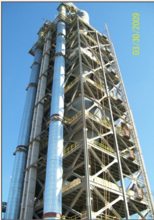
Pre-heater tower and stack
