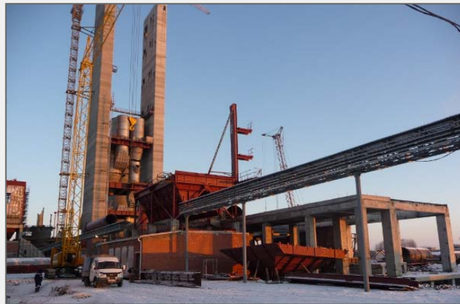
Tower and kiln line
